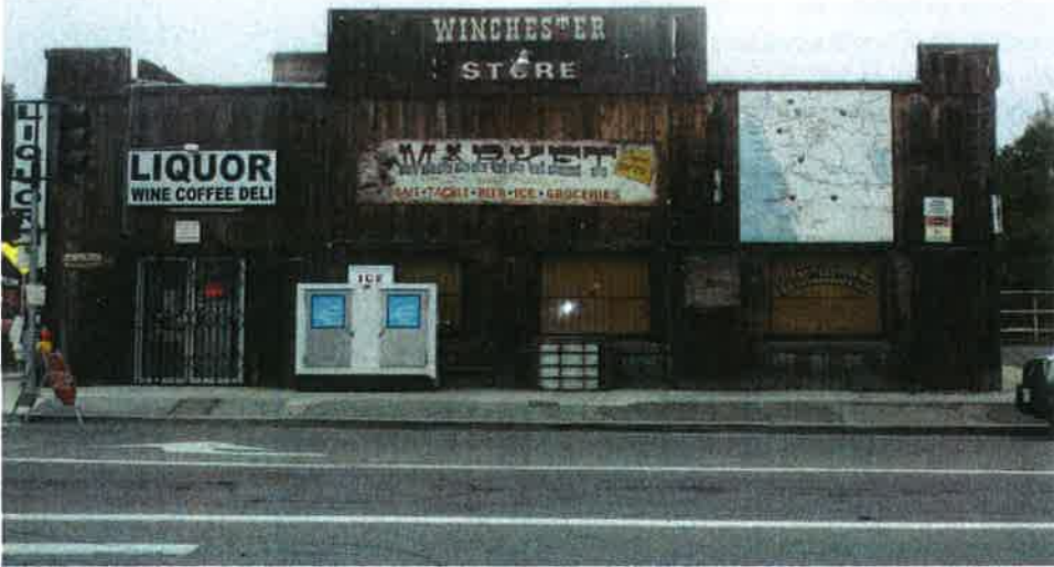
Existing Commercial Building
