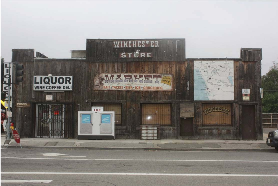
Existing Commercial Building
