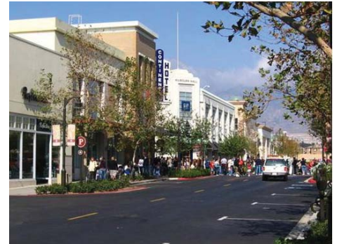
Commercial Development Outside of Downtown Core
